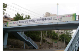
<Seoul Art High School Overpass>
